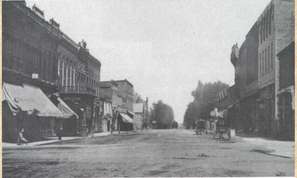
Downtown Clay City, IN, looking north. Nov 28, 1910
